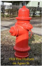
Owatonna Public Utilities maintains 1238 public and 113 private fire hydrants within the city limits. The oldest fire hydrant is dated 1924 and is located on Agnes St. The average cost of a new fire hydrant is \$2,500. Maintenance of fire hydrants consists of painting and annual flushing. Every hydrant is flushed yearly.
